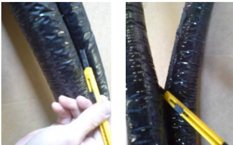
Cut around the insulation to reveal the pipe, this is then cut using a pipe cutter.
