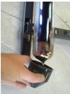
Push copper tip of the heat pipe into manifold (don't worry if tip is slightly bent, the copper is quite soft). The opened jubilee clip is threaded through the slots in the frame's lower rail and lightly tightened around the rubber end cap. If using a cordless driver with an 8mm bit, remember to turn the torque setting down to prevent cracking the tube. Repeat until all the tubes are in.
