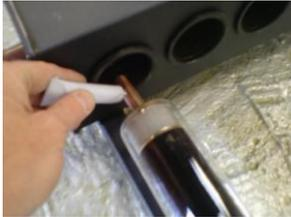
Next, Put rubber end caps on tube – it is often easier to wipe a little washing up liquid around the top and the bottom ends of the glass tubes to ease fitting.
