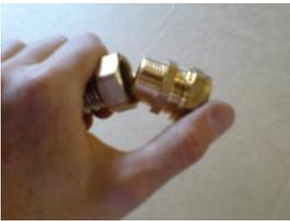
4. Unscrew the fitting, insert the washer, reconnect the fitting and tighten.
