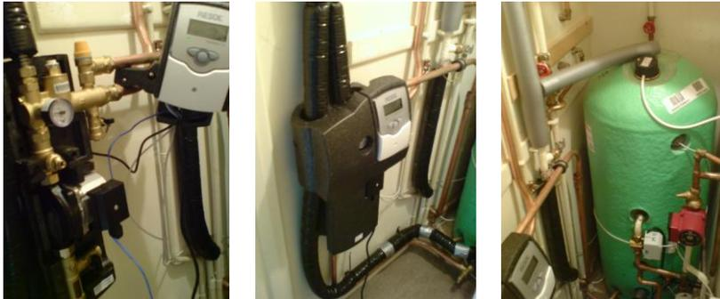
Connect the return DN16 2-in-2 pipe (the one carrying fluid back to the collector) to the top connection of the pump station using a PAW self seal nipple and the back nut – black rubber seal facing towards the pump station.
